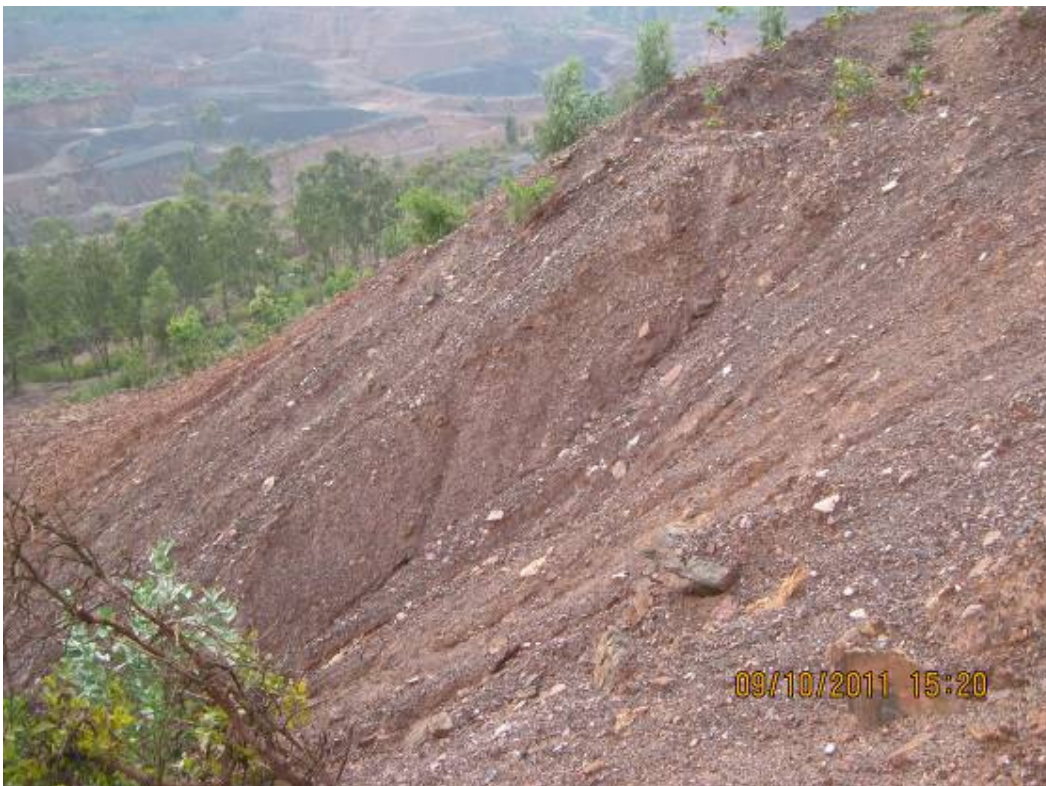
Deep gully formation and erosion of OB dump of Hanuman mines of Tumkur
