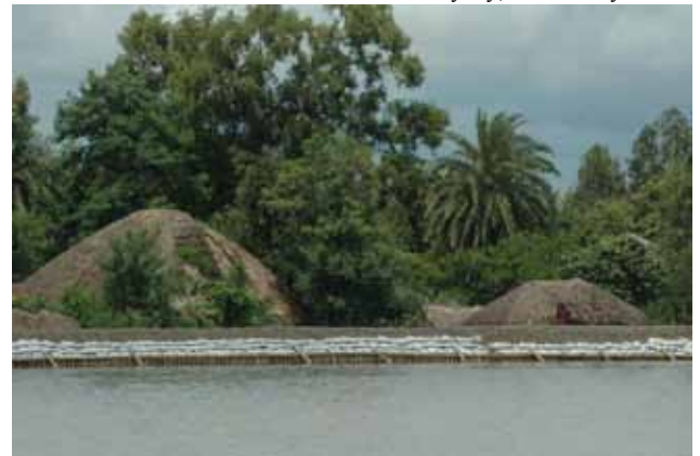
There are 54 populated islands in Sundarban facing High Tide twice a day – nearly 3500 km long embankment protect 54 islands from the threat of flood everyday, twice a day
