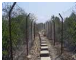
Progress in Construction for Sunderban site
