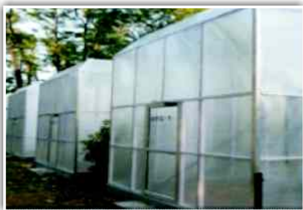
OTC's facility developed at FRI, Dehradun
