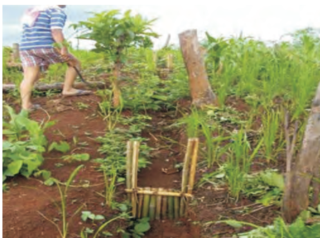
Bamboo Check Gate for Soil Conservation
