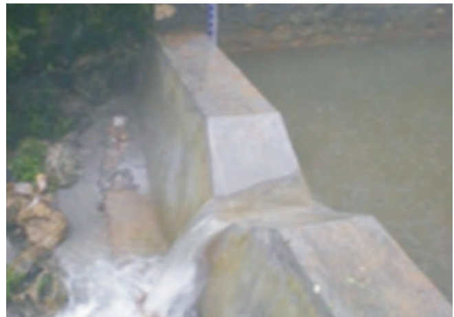
Weir at Site
